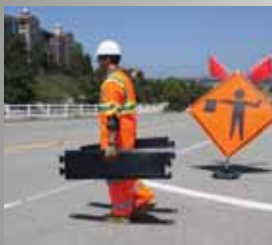
One worker can quickly and easily deploy a Traffix Alert zone in minutes, without additional tools, minimizing exposure to traffic.
